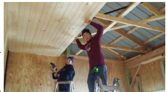
The Ceiling Is Going In!
